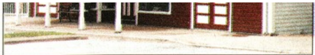
Mitch Kloorfain / chief photographer Stuart Heritage Museum, located at the end of Flagler Avenue in downtown Stuart, is a small wood frame building built in 1901. It is one of the last of its kind remaining on the southeast coast of Florida.
